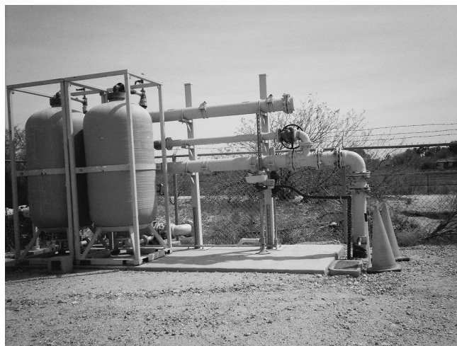
Pictured above are the Hub No. 1 Treatment System Vessels that remove arsenic, a naturally-occurring mineral in the Southwest, and ensure compliance with the Safe Drinking Water Act.
