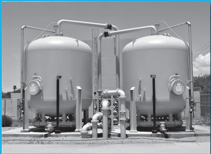
*Metro Water District's South Shannon Treatment System (pictured above) pumps water through two vessels filled with granular activated carbon (GAC) which is effective at removing PFAS. ♡*
