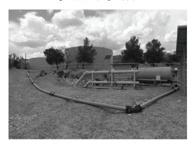
Pictured above is a temporary "highline" at Metro Hub Reservoir. This bypass method keeps customers in water while repairs are made.
