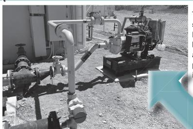
To ensure resilient and reliable water service in the Metro Southwest - E&T service area, a diesel powered booster pump was recently installed at the E&T 22 well site. This booster pump will help minimize water service interruptions during power outages.
