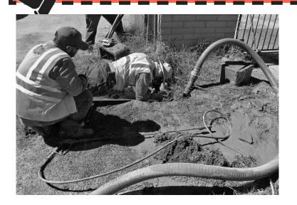
Pictured is Eric Gaytan, Utility Technician II, (right) and Albert Westrope, Utility Technician II, (left) working to repair a failed polybutylene waterline in the Metro Southwest - Diablo Village service area. The District's Utility Team performs proactive and emergency maintenance activities to ensure deliveries of safe and reliable water to District customers.
