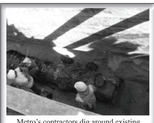
Metro's contractors dig around existing utilities to relocate water line. They must work in deep, tight trenches to successfully relocate water mains.
