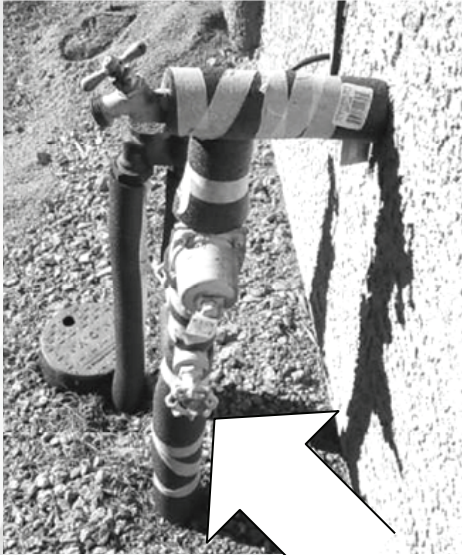
HOUSE VALVE / SHUT-OFF VALVE
