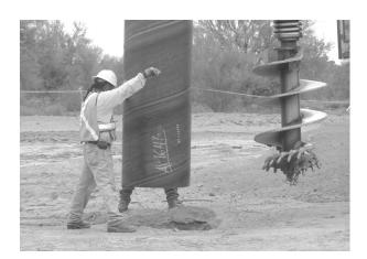
The Magee Trail well is one of Metro Water's newest wells. Shown left, the drilling contractor (Arizona Beeman Drilling) began the process of drilling the new well, which ultimately reached 1,000 feet, double the depth of the groundwater table.
