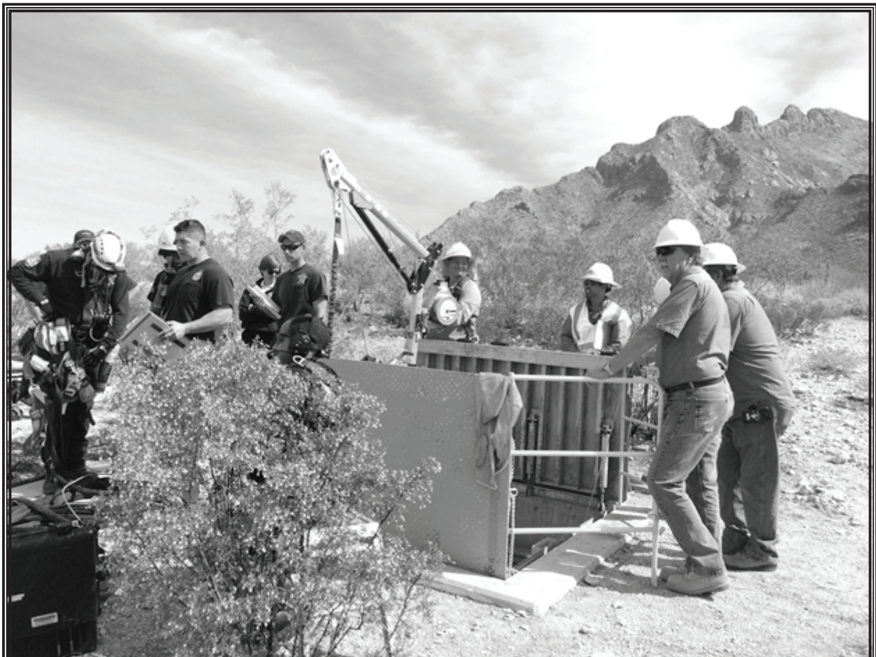
From April 5th to 7th, Metro Water staff partnered with Northwest Fire and Golder Ranch Fire on a joint confined space rescue training at the District's James M. Tripp Reservoir. This mutually beneficial training honed first responders' confined space recovery skills and provided insight on how to respond to emergencies at District facilities.
