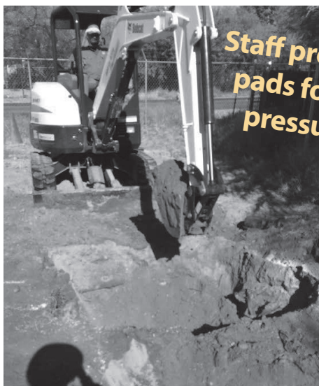
The old E&T 22 pressure tank being removed.
