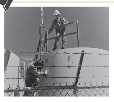
Prior to installing a new internal coating to one of the E&T Storage Tanks Cory Bott, Utility Supervisor, and Austin Bott, Utility Technician I (pictured at left) installed a safety railing on the storage tank.
