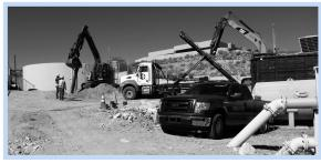
Old Nogales Highway Waterline Replacement. This project located in the Metro Southwest – E&T service area is needed due to continued breaks occurring in the existing waterline. Once completed, the newly constructed waterline will improve reliability and minimize service outages. Another key benefit to this project is the cost savings associated with the elimination of numerous emergency call-outs necessary for repairs.
